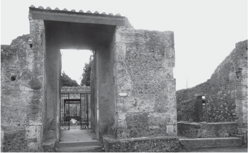
Plate 1 (CD 4): Casa di D. Octavius Quartio (II 2,2; PPM III 43): doorway, client benches, view into atrium (2); to the viewer's right from the doorway, a thermopolium (1) that is both open to the street and also has back door into atrium (2) of the house.
