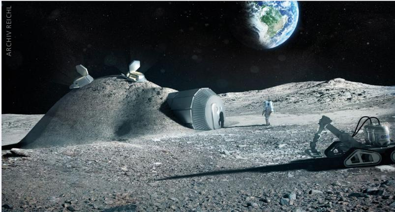
In order to protect the habitat from radiation it has to be covered with a blanket of two to three meters of lunar regolith.
