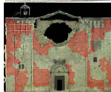
Thermographic mosaics of the detached masonry of the façade
